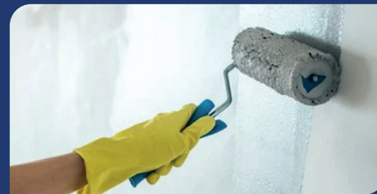
Carpentry, masonry and painting works
